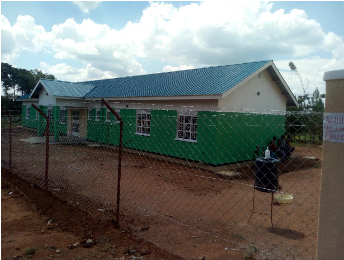
Newly constructed and fenced maternity wing in Buwumba Health Center II. The community contributed labour and cash of approximately $270
